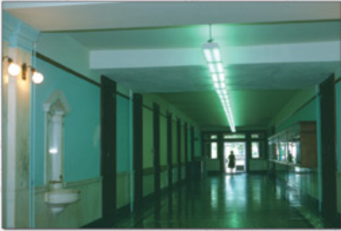
Over the years, the capitol was updated and modernized. More offices were created by adding walls. Fluorescent lights went in. Ornate decoration disappeared under coats of paint.
