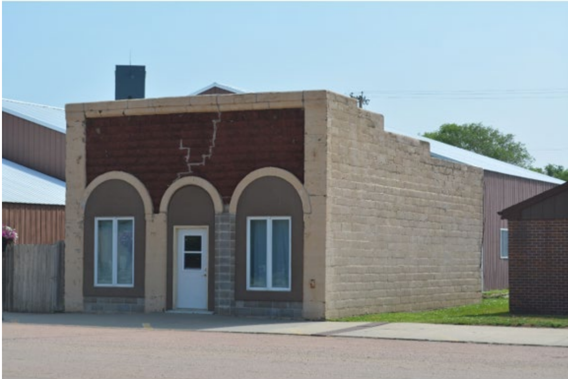
SD_CharlesMixCounty_GeddesHistoricDistrictAdditionalDocumentation_0007. Looking East at the 300 Block Main Street (east side).
