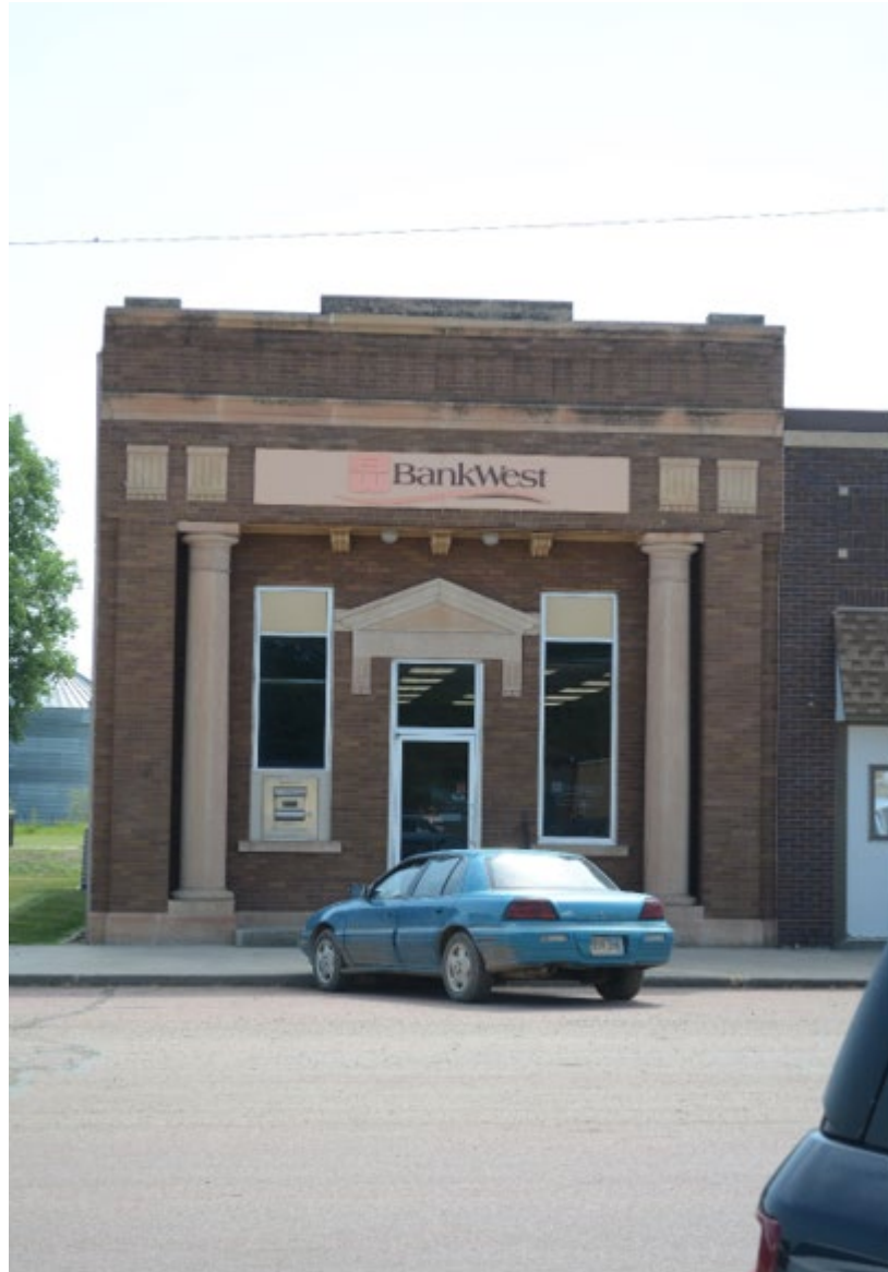
SD_CharlesMixCounty_GeddesHistoricDistrictAdditionalDocumentation_0006. Looking East at 218 Main Street.
