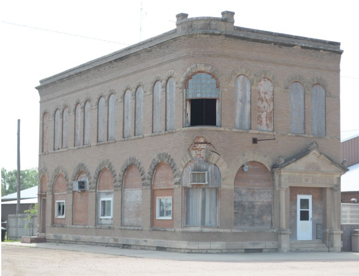
300 Main. Bank of Geddes. C.W. Pratt constructed this building in 1908 utilizing pressed brick, Bedford limestone, and variegated marble on the interior. The bank closed around 1927. Subsequent business included Mrs. Miller's Ladies Hat Shoppe, Drs. Privet and Klare, the Beauty Shop, and Red Oaks Bar.
