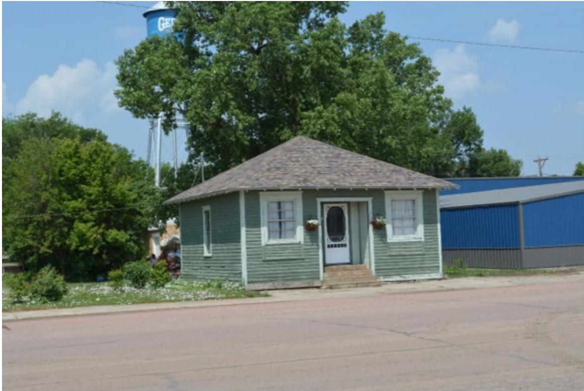
SD_CharlesMixCounty_GeddesHistoricDistrictAdditionalDocumentation_0011. Looking West at 409 Main Street.
