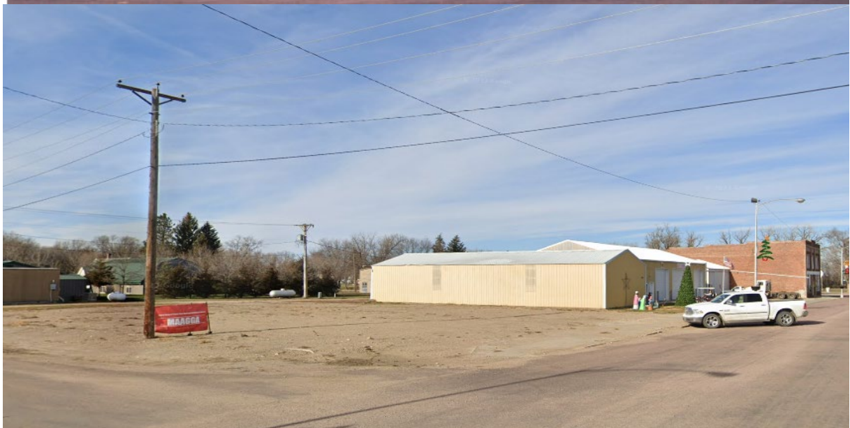
200 Block of Main Ave (west side). Padley Hotel and false-fronts buildings circa 1973 (top) and today (bottom). (Top photo courtesy South Dakota State Archives)
