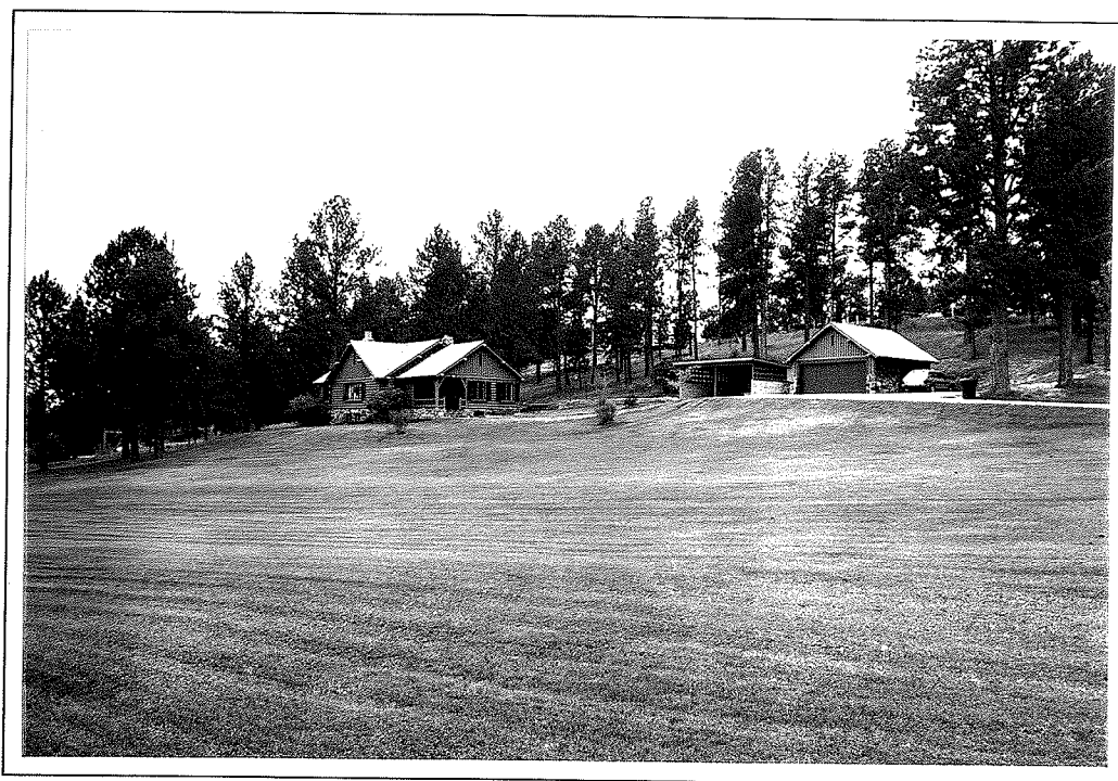
Figure 34. Forest Service ranger's dwelling and garage, Custer. (Dennis, 1997)
