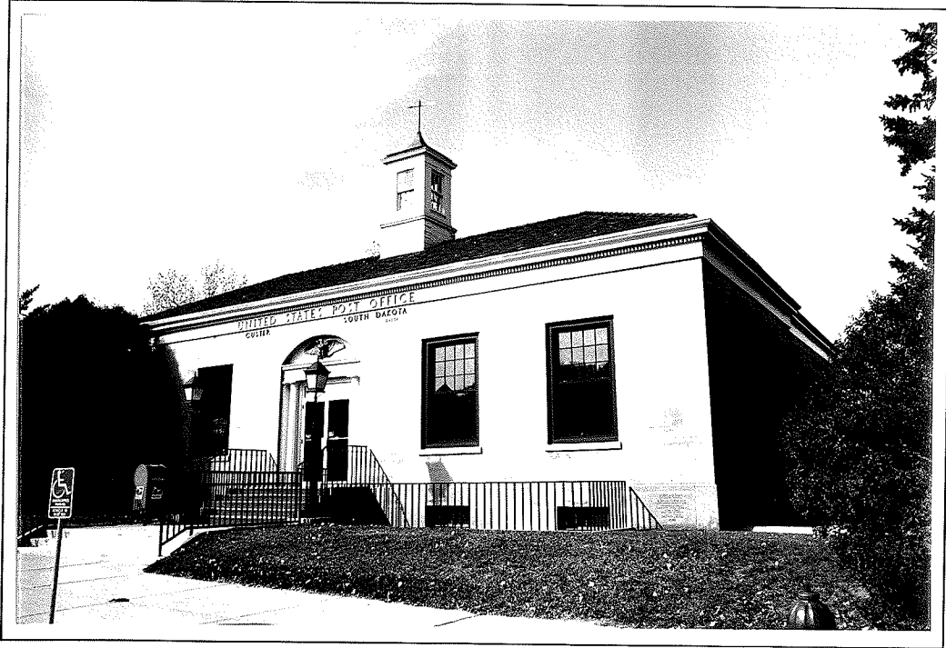
Figure 22. Post Office, Custer. (Dennis, 1997)
