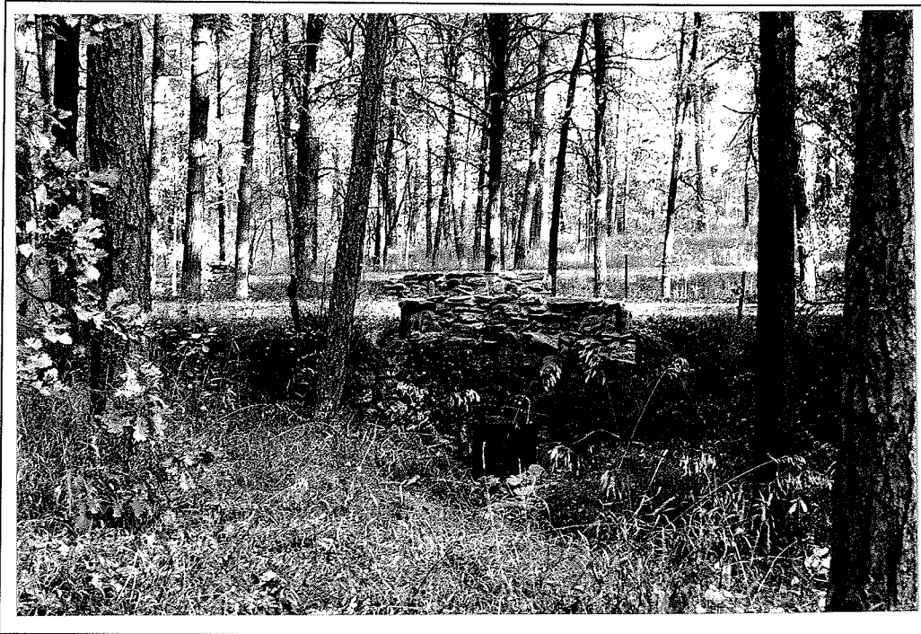
Figure 51. Stone culvert at Grizzly Bear picnic ground, Black Hills. (Dennis, 1997)
