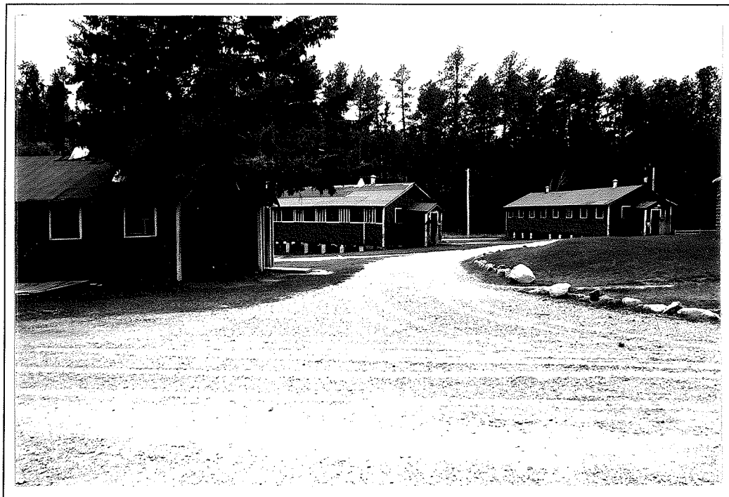
Figure 50. Three of the remaining barracks buildings, Camp Lodge, Custer State Park. (Dennis, 1997)
