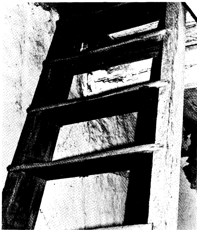
Fig. 42. Pictured here is the ladder to the loft at the Ziegler house-barn. Sturdy and well-constructed, these ladders with mortised steps are found commonly in German-Russian homes.
