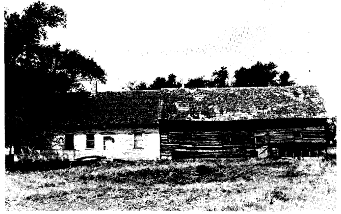
Fig. 64. Built entirely of wood is the Joe P. Gross house-barn. Note the location of the windows and door.
