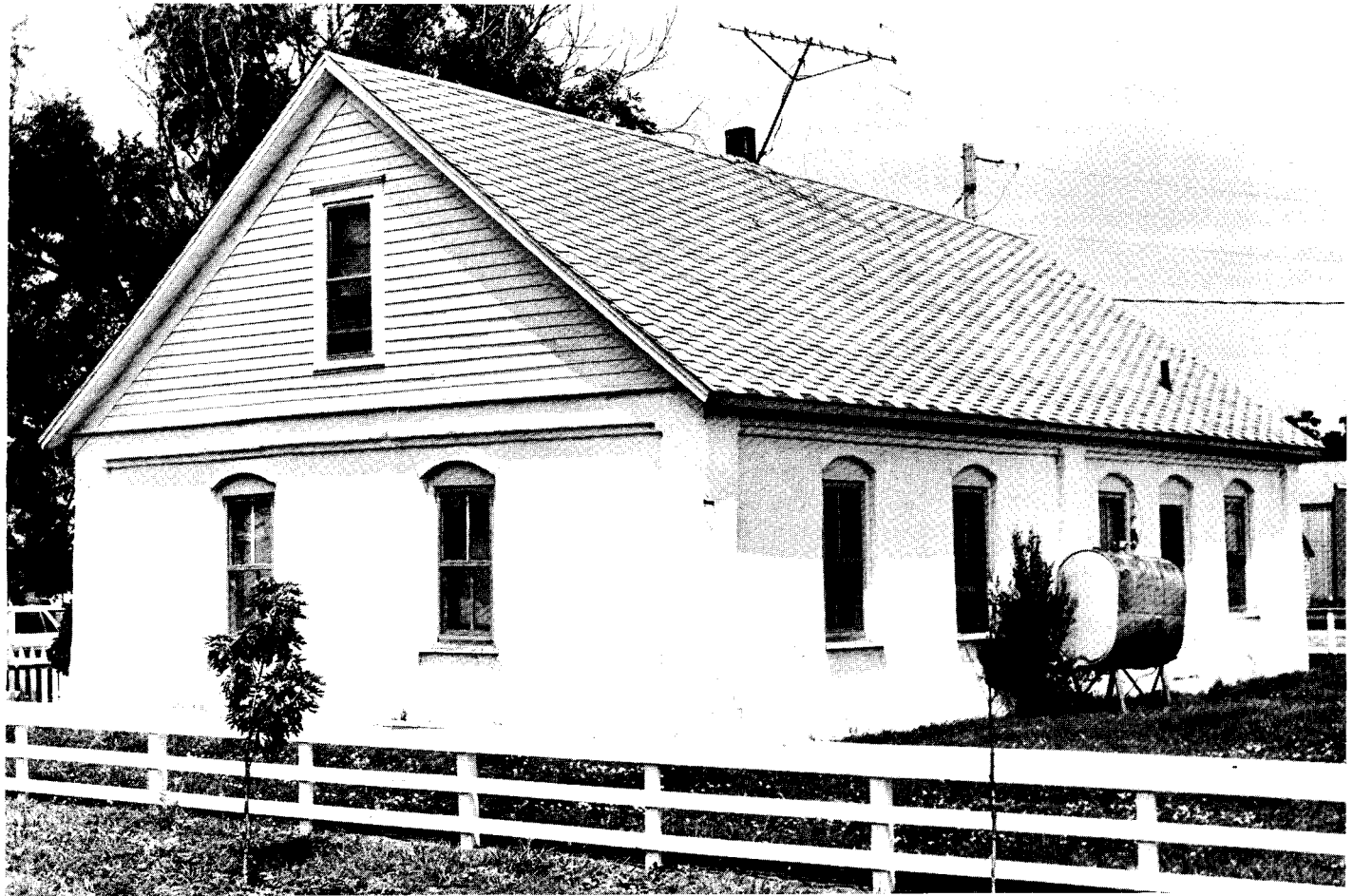
Fig. 65. The Paul Pullman house is built of locally-made, kiln-fired brick. Arched windows, whitewash and pilasters are characteristics found in Ukrainian houses.
