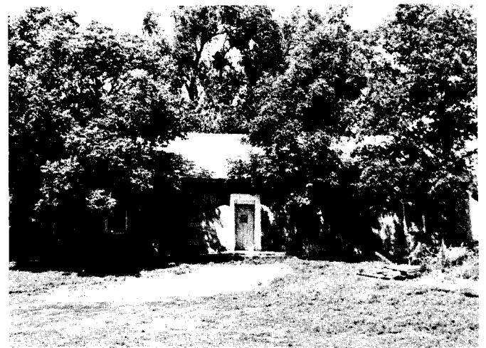
Fig. 44. The east elevation is shown in this photograph of the Phillip Lang house.
