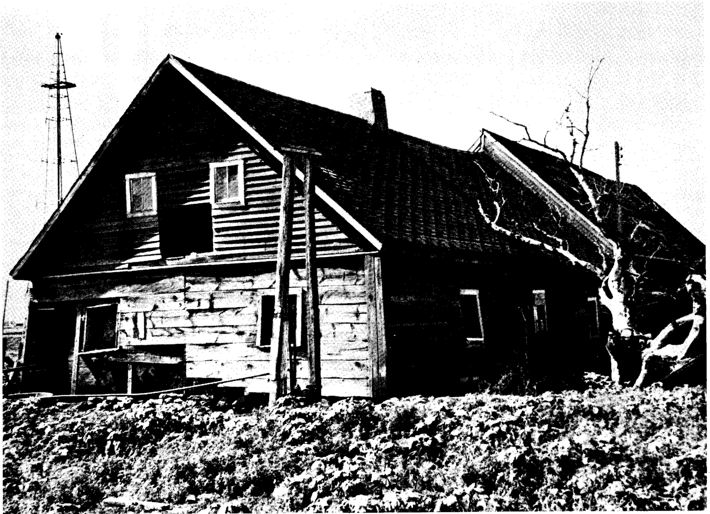
Fig. 11. The southeast elevation of the Kleinsasser house-barn is shown here.
