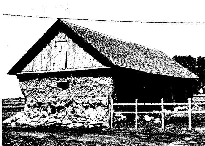
Fig. 61. This rammed earth barn similar to the Schmidt house displays the various layers of the clay in the wall.
