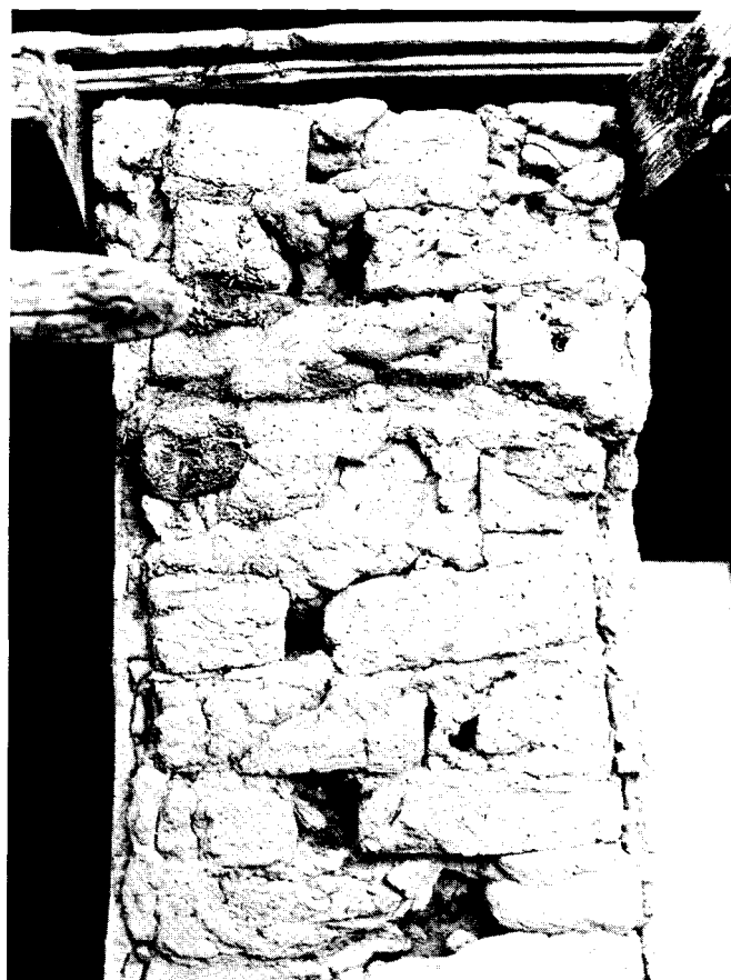
Fig. 49. A section of a wall at the Rademacher house shows the batsa brick, clay mortar and a thin veneer of clay and whitewash.
