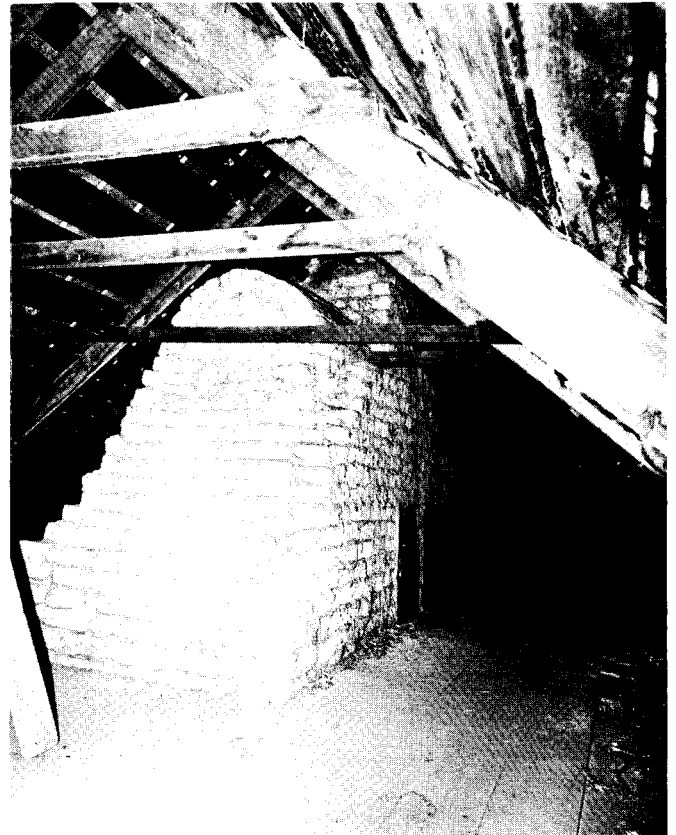
Fig. 53. Martin Grosz, the grandfather of the present owner, built this decorative arch on this batsa chimney. This massive chimney has a small wooden door on one side. The meat to be smoked was placed in the chimney through the door.
