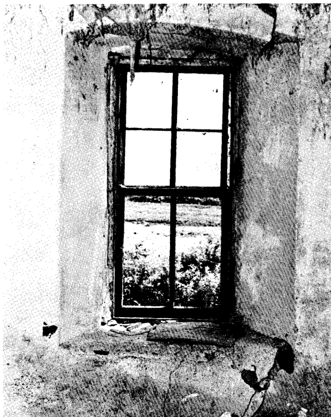
Fig. 39. An interior view of the previous window shows clearly a continuation of the arch. Note the wall thickness and angled window opening which takes full advantage of solar heating.
