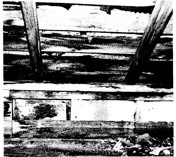
Fig. 25. This detail taken in the loft shows batsa brick infill between vertical wall studs; horizontal tongue and groove boards partially cover the bottom of the bricks. The distance between each 2" x 4" stud is 16".
