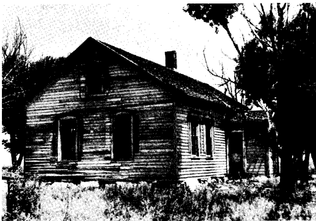
Fig. 24. The frame and batsa brick Rempfer-Wagner house in Yankton County is pictured here.
