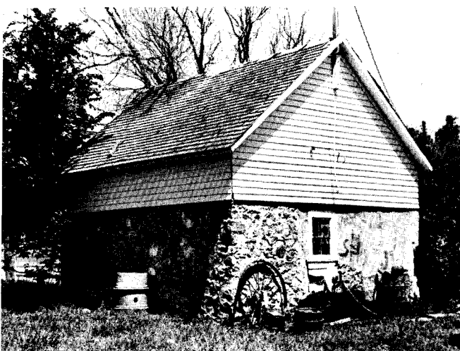
Fig. 63. Pictured here is the Heckenlaible shed.
