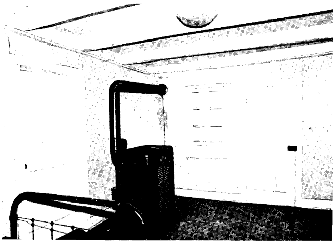
Fig. 34. Although no evidence of a furnace/bake oven was found at Site 8, the same general spacing of doors and the location of a recessed cupboard indicate a typical German-Russian house with furnace/bake oven. Note the chamfer on the exposed stringers.
