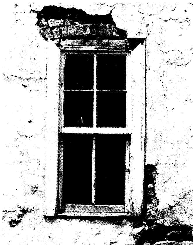
Fig. 38. What appears to be a completely stone masonry wall in the Sedlacek house actually contains a brick jack arch above the double-hung sash window.
