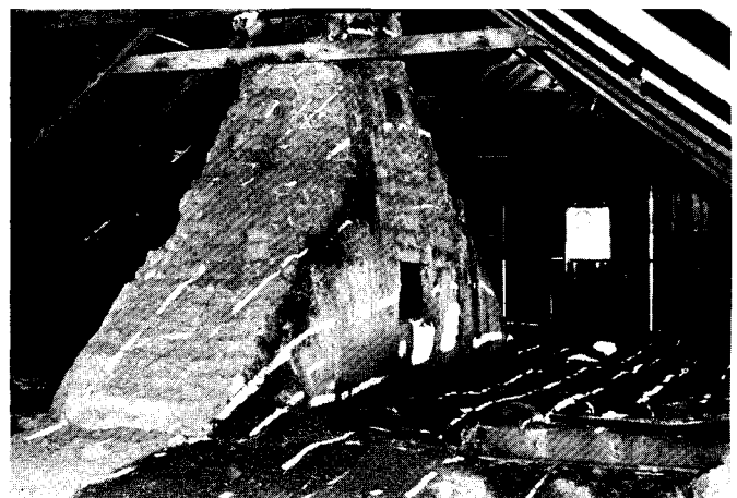
Fig. 60. This batsa brick chimney is very similar to the Grosz chimney at Site 14. Note the small meat smoking opening near the loft floor.
