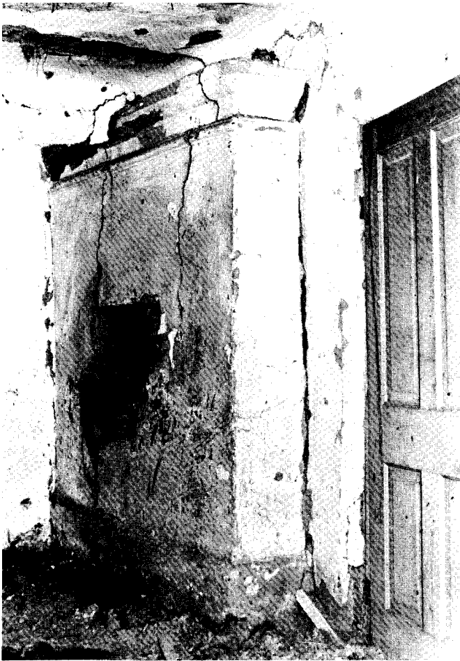
Fig. 59. Pictured here are the crumbling remains of the furnace/bake oven at the Schmidt house. Note the clay mold at the top of the oven.
