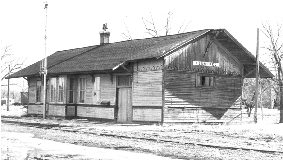
Figure 23. The Milwaukee Road's Kennebec depot is a quintessential implementation of a standardized wood-framed depot design (State Historic Preservation Office photo).
