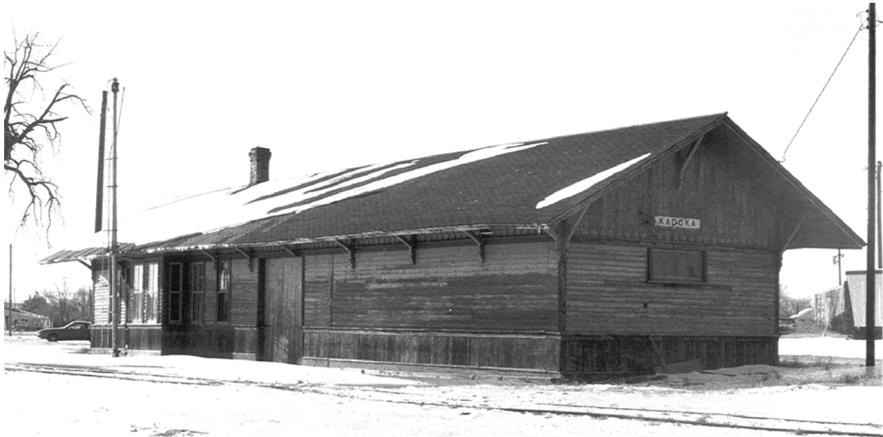
Figure 20. A trackside view of the Milwaukee Road's combination depot in Kadoka (State Historic Preservation Office photo).
