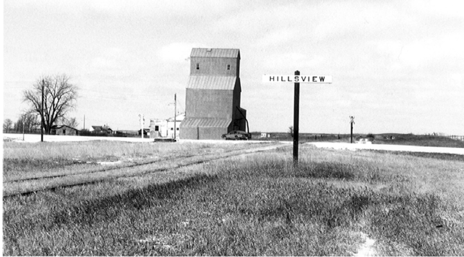
Figure 1. The barely-discernable rails of a Milwaukee Road branch line pass a lonely grain elevator at Hillsview, South Dakota (State Historic Preservation Office photo).
