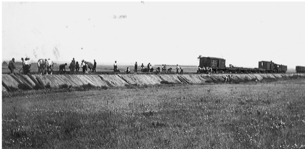
Figure 6. Tracklaying crews working to complete the Milwaukee Road branch line to Wessington Springs, 1903 (South Dakota State Archives photo).
