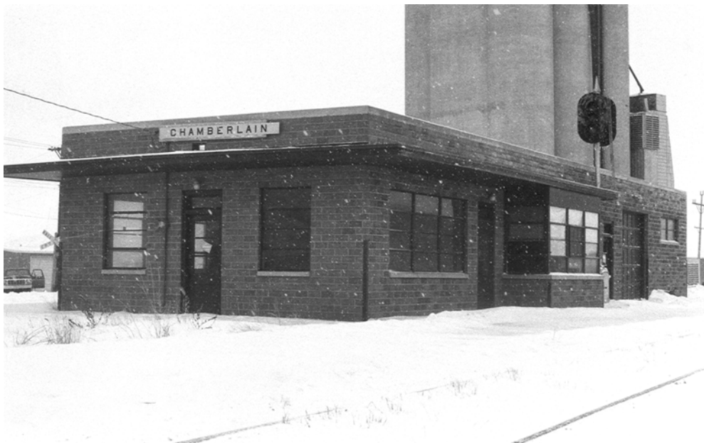
Figure 40. A 1970s view of the Milwaukee Road depot in Chamberlain, now the headquarters building of the Dakota Southern (State Historic Preservation Office photo).
