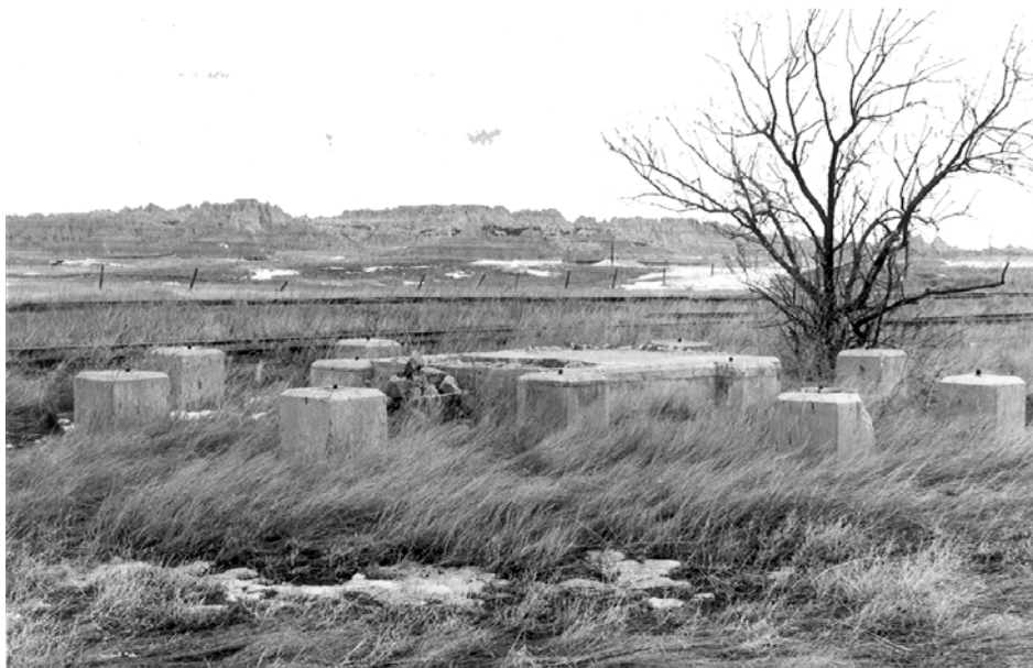
Figure 39. The footings of a former water tower along the Milwaukee line through Interior suggest the possibility of a Criterion "D" site in the area (State Historic Preservation Office photo).
