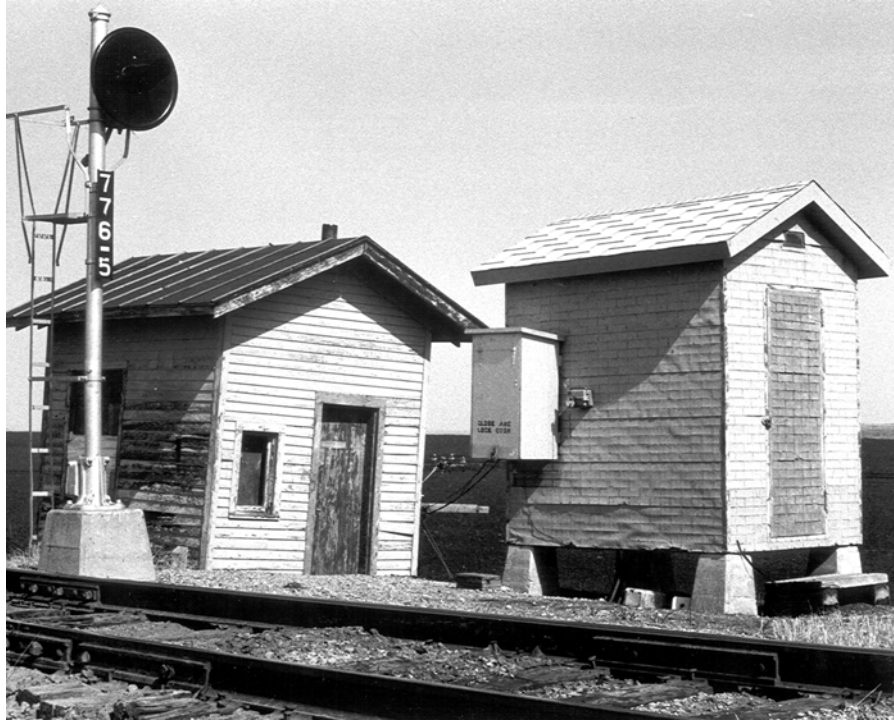
Figure 34. An electric color-light signal, switchman's shanty, and telephone box, along the Milwaukee Road in Walworth County (State Historic Preservation Office photo).
