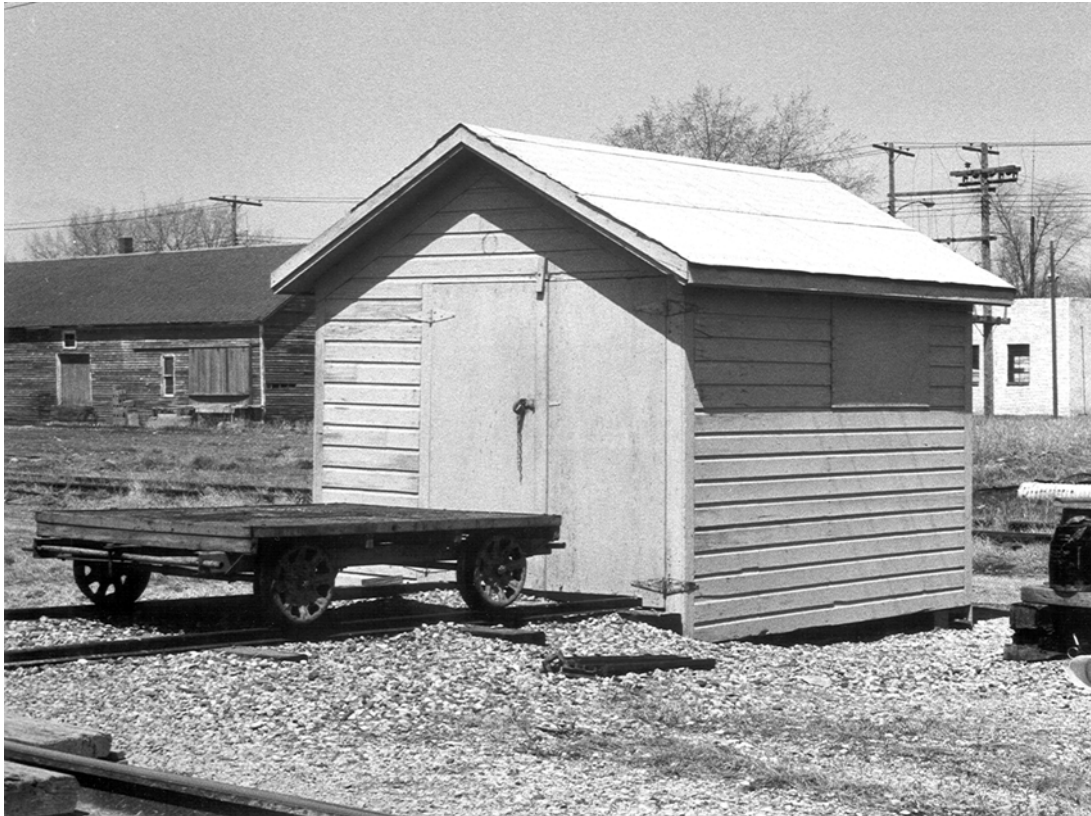
Figure 30. A small handcar house at Ipswich, on the Milwaukee Road main line (State Historic Preservation Office photo).
