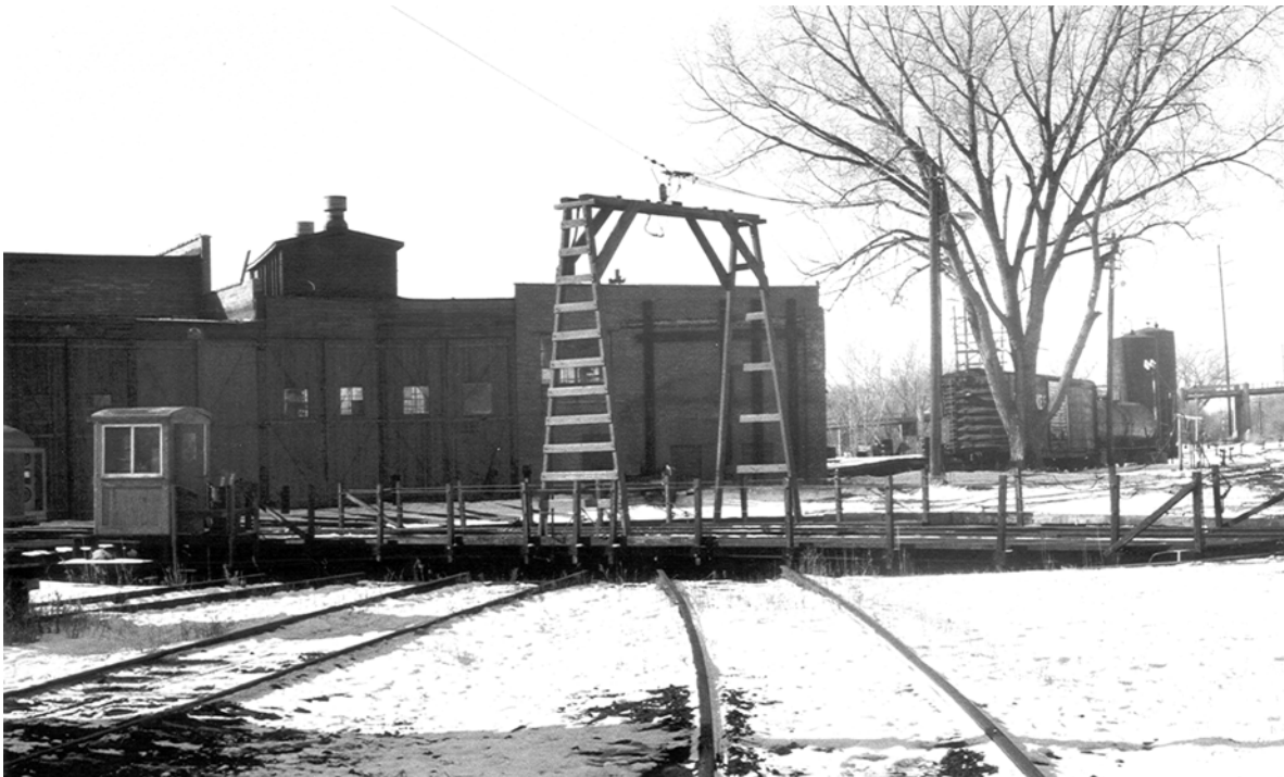
Figure 26. The turntable servicing the Milwaukee Road's Mitchell roundhouse (State Historic Preservation Office photo).
