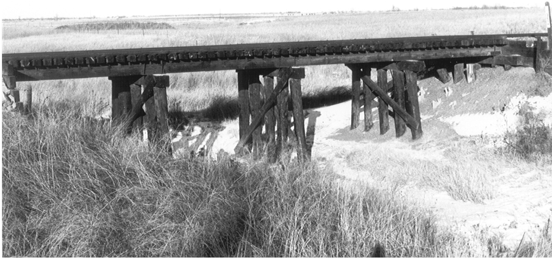
Figure 31. A typical example, from the Milwaukee Road, of a small timber trestle (State Historic Preservation Office photo).
