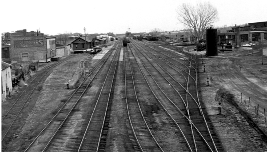
Figure 37. A 1970s view of the Milwaukee Road yards in Mitchell (State Historic Preservation Office photo).
