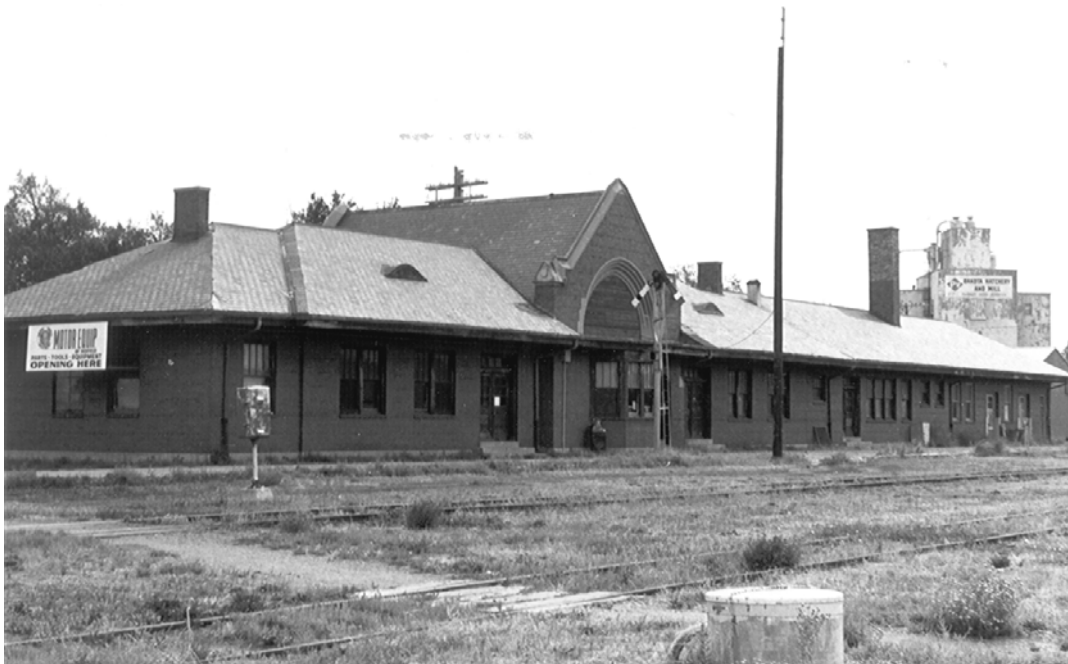
Figure 17. The Chicago & North Western station in Redfield is a fine example of a mid-sized masonry depot building (State Historic Preservation Office photo).
