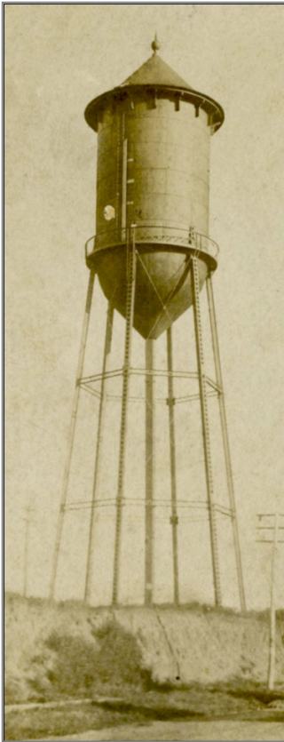
FIGURE 1. SIOUX FALLS WATER TOWER NO. 2, 1896 (Courtesy Siouxland Heritage Museums)
