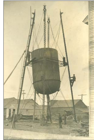
FIGURE 4. WATER TOWER UNDER CONSTRUCTION IN RAPID CITY (Courtesy State Archives of the South Dakota State Historical Society)
