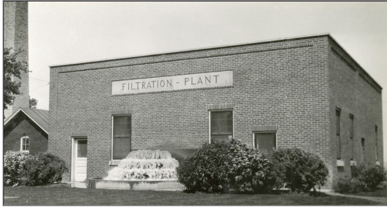
FIGURE 27. FILTRATION PLANT, LAKE KAMPESKA, WATERTOWN (Courtesy State Archives of the South Dakota State Historical Society)
