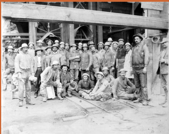
Crew at the Holy Terror Mine, Keystone, S.D., 1900- 1905. SD State Archives
