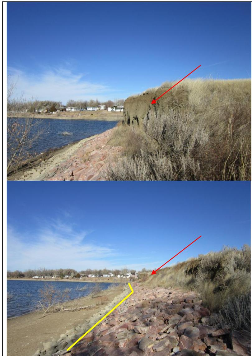
Figure 112. Close-up (top) and wide-angle view (bottom) of cut bank and riprap shoreline below 39FA65 in November 2011. Facing north. Note the 2011 high water mark at approximately 2,187 feet amsl (yellow line in bottom frame) and the start of revegetation. Red arrow identifies the cut bank.
