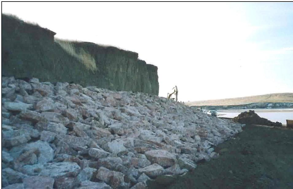
Figure 111. Revetment profile from the toe to the catch point when the work was nearly completed with a catch point at 3,192.0 feet. The exposed surface of the riprap on the shoreline is at 3,186.0 feet.
