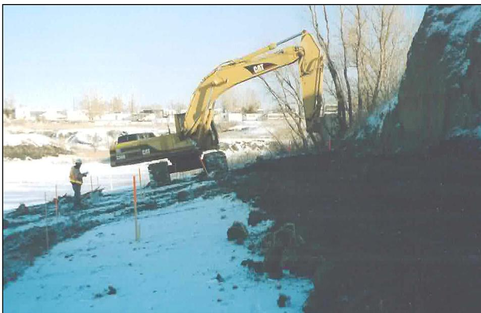
Figure 109. Debris clearing and preparation for excavation of the toe trench.
