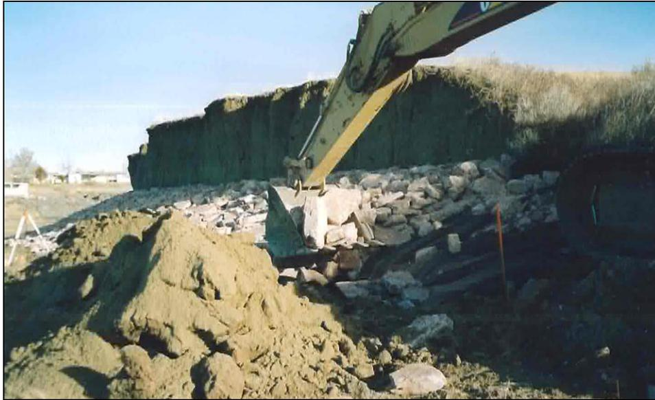
Figure 110. Riprap placed over granular fill base and fabric.
