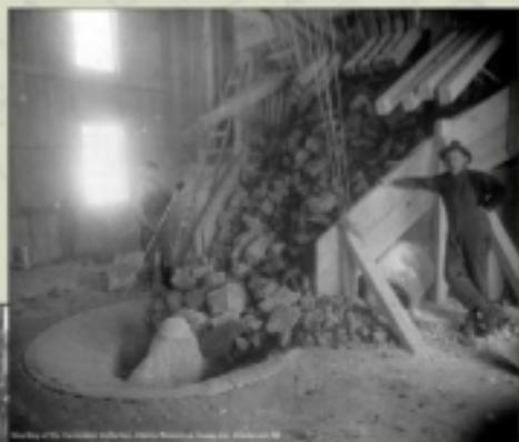
*On the surface, ore crushers smashed the rock into 1/2-inch pebbles.*
