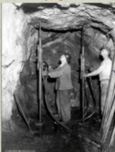
Drilling overhead, ca. 1946. Miners dubbed the overhead drills "widow makers." Falling rock caused more deaths than anything else in the mines.
