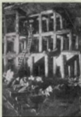
Square-set timbers shored up a stope at Homestake, ca. 1906. Workers could move ore through the chutes to cars on the ground level.
