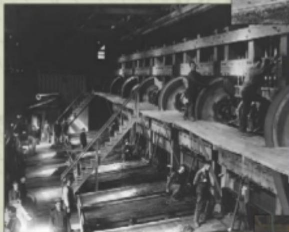
*Homestake's cyanide plant, ca. 1920. Miners used cyanide, mercury, and other dangerous chemicals to process gold. Chemical reactions filled the air, often making workers sick. Spills into local streams could be disastrous. A cyanide overflow in 1901 killed thousands of trout in Spearfish Creek.*
