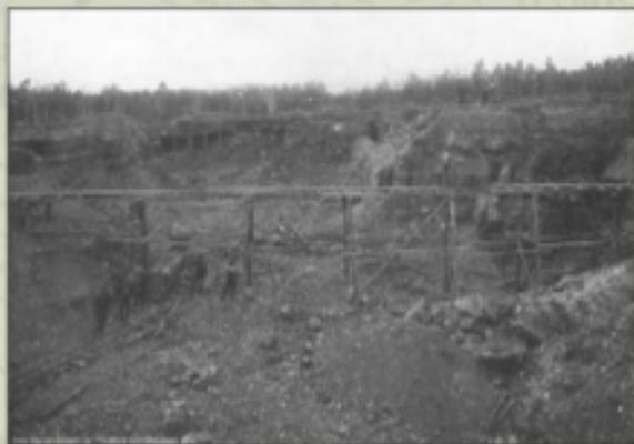
*The Wasp No. 2 Mine near Terry, pictured in 1904, used open-cut mining. It moved rock with dynamite and surface equipment instead of building an underground system of shafts.*
