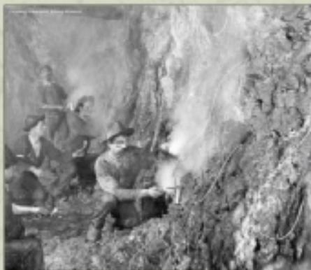
*Lighting fuses for a mine blast, ca. 1900. Miners used varied lengths of fuse to get the right blast sequence. This meant lighting more than one fuse at a time, a dangerous practice. Automated blasting caps later made this job safer.*
