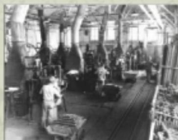
*Homestake Mine's drill-sharpening shop, ca. 1960. To cut through solid rock, miners needed freshly sharpened drill bits each day.*
