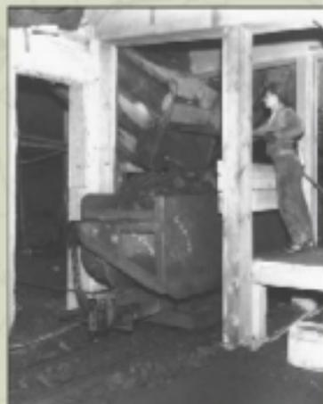
Filling an ore car in Homestake with a drawing chute, 1960.
