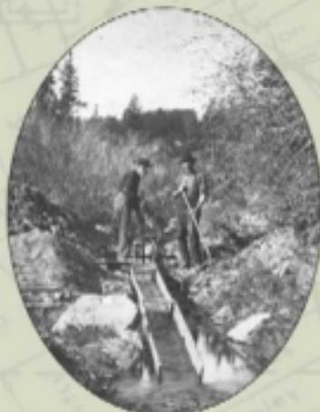
*Miners working a sluice, ca. 1876. Surface or placer mining uncovered minerals like gold on the earth's surface. One or two people could run a placer mine with little equipment.*
