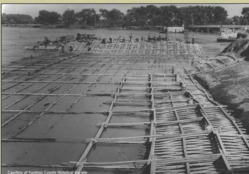
POWs installed riprap along the Missouri River near Yankton, ca. 1945.
