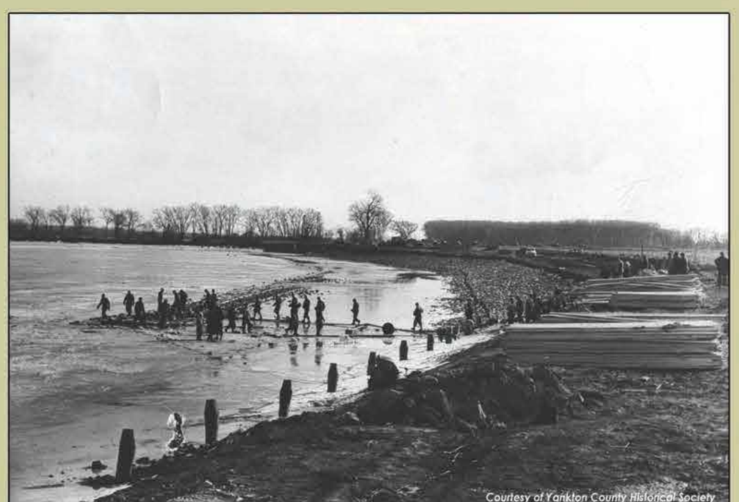
POWs installed riprap along the Missouri River near Yankton, ca. 1945.
