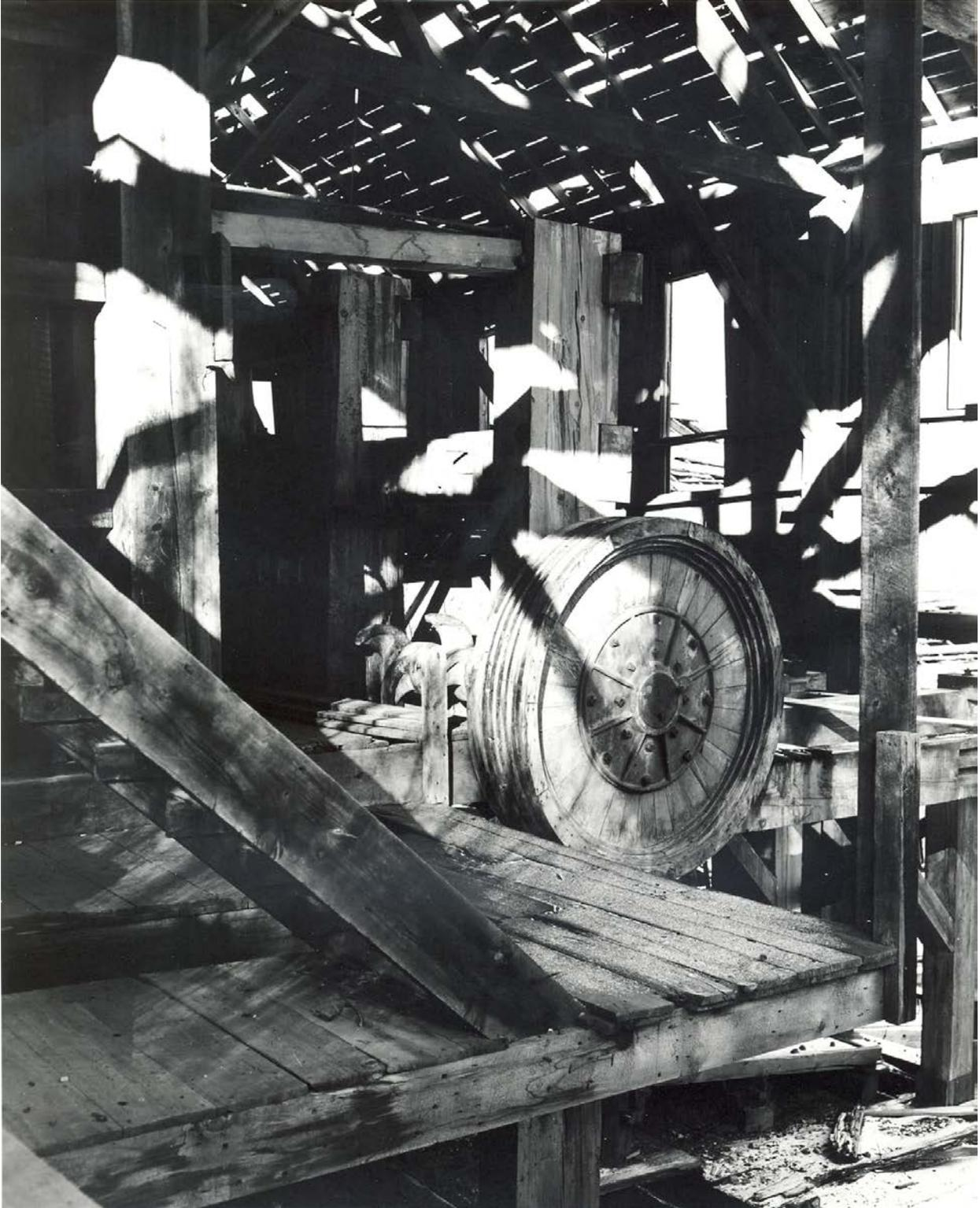
Figure 3.75: Wheel and cam on a stamp at Standby Mine near Rochford. Courtesy South Dakota State Historical Society.
