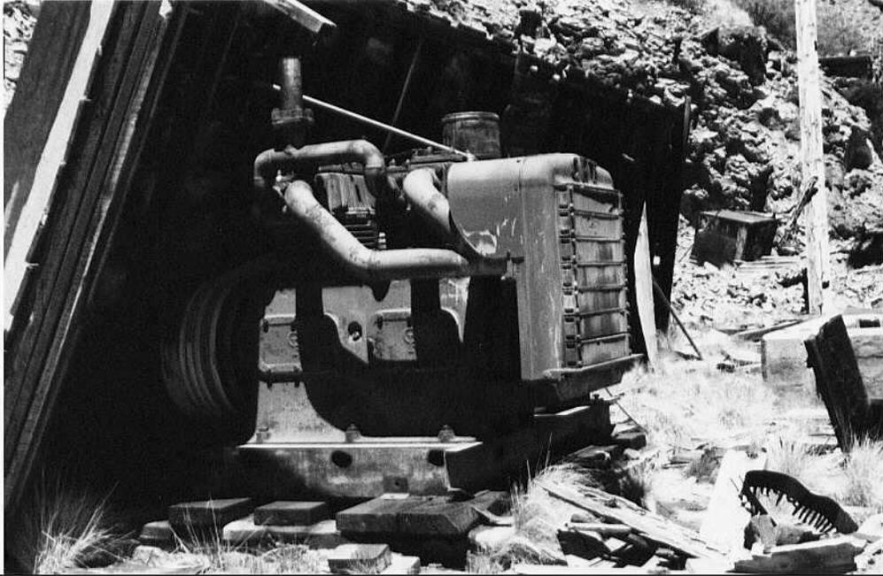
Figure 3.43: The V-cylinder compressor, similar to a large engine, became one of the most popular compressor types during the 1930s. Note the foundation. Source: Twitty, 2002:274.
