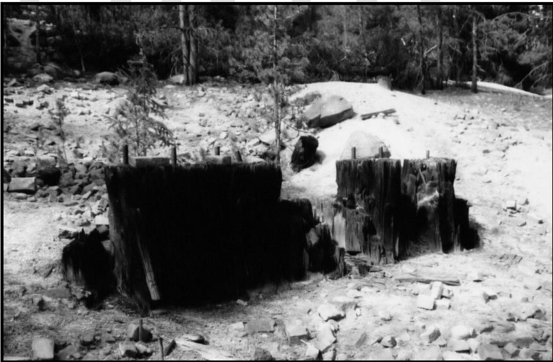
Figure 3.80: When a stamp battery was dismantled, the pedestals for the cast iron battery boxes were often left in place. The pedestals consist of timbers on-end and feature anchor bolts on top, and each is around 2 feet wide, 3 feet high, and 5 feet long. Source: Eric Twitty.
