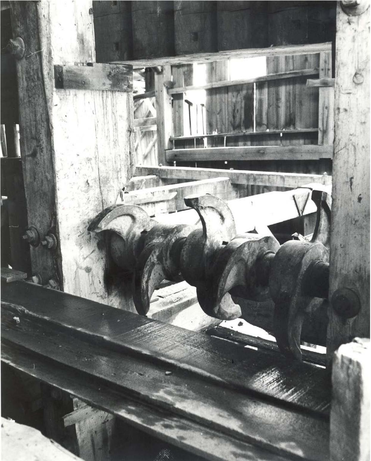
Figure 3.76: Close up of cam at Standby Mine in Rochford. Courtesy South Dakota State Historical Society.
