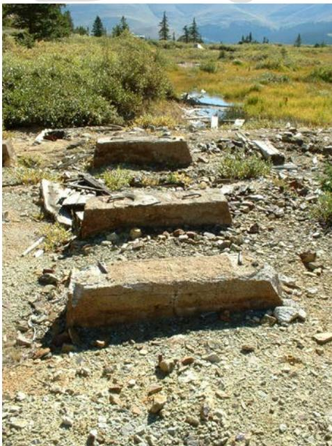
Figure 3.91: Vibrating tables like the one in Figure 3.69 below were anchored to foundations of three concrete or timber footers, often 5 feet wide and 15 feet long. Source: Eric Twitty.
