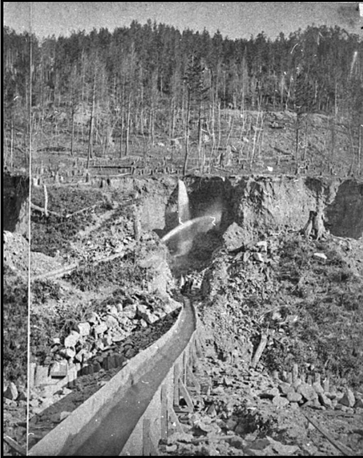
Figure 3.4: Hydraulic mining utilized jets of water to erode thick gravel banks, and ditch flows to wash the material through lengthy sluices. In 1878, this Deadwood mine was a microcosm of hydraulic mining. A monitor emits an arced jet against a precipitous cut-bank of gravel, and a waterfall from a ditch carries the liquefied gravel into the sluice. Courtesy of the State Archives of South Dakota Historical Society.
