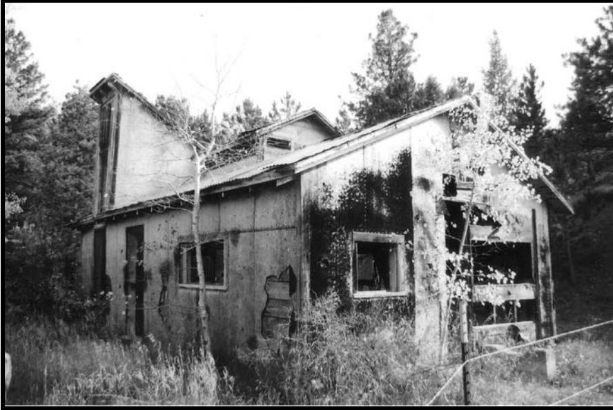
Figure 3.33: In this hoist house example dating to the 1930s, the left roofline features an angled cupola for the hoist cable, which ascended to a headframe left and out of view. Source: Eric Twitty.
