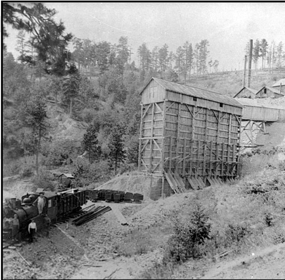
Figure 3.55: The Hoodoo Mine had a sloped floor ore bin characteristic of heavy production. Miners input ore via the covered trestle at top, and freighters extracted the payrock through the chutes at bottom for shipment to a mill. Today, such bins can manifest as log and timber foundations, structural debris, and a platform. Courtesy of the State Archives of South Dakota Historical Society.
