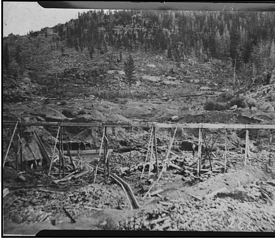
Figure 3.3: The undated photo illustrates a typical stream placer mine in the Black Hills. Characteristic are piles of tailings, debris, log dams, and the sluices curving through the piles. A diversion flume crosses the foreground and carries water to another mine. Today, such a site may include the tailings, the dams, and archaeological evidence of the structures. Courtesy of the State Archives of South Dakota Historical Society.
