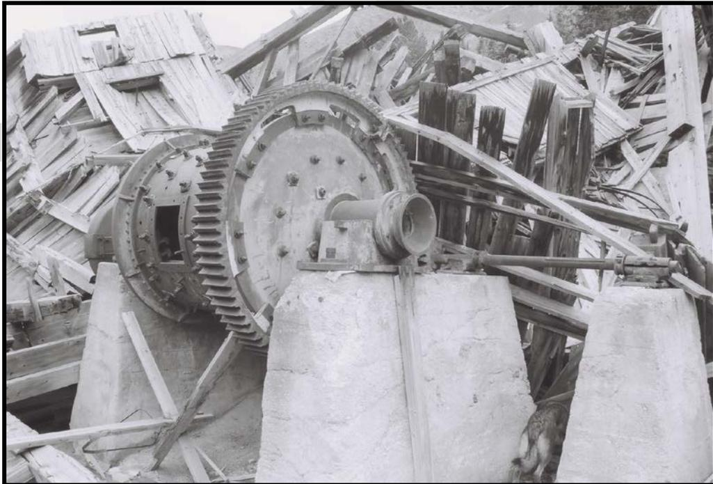
Figure 3.84: The ball mill performed similar to the rod mill above. The difference was that steel balls tumbled in the chamber and ground ore to a slurry. Note the concrete foundation, distinct in footprint. Source: Eric Twitty.
