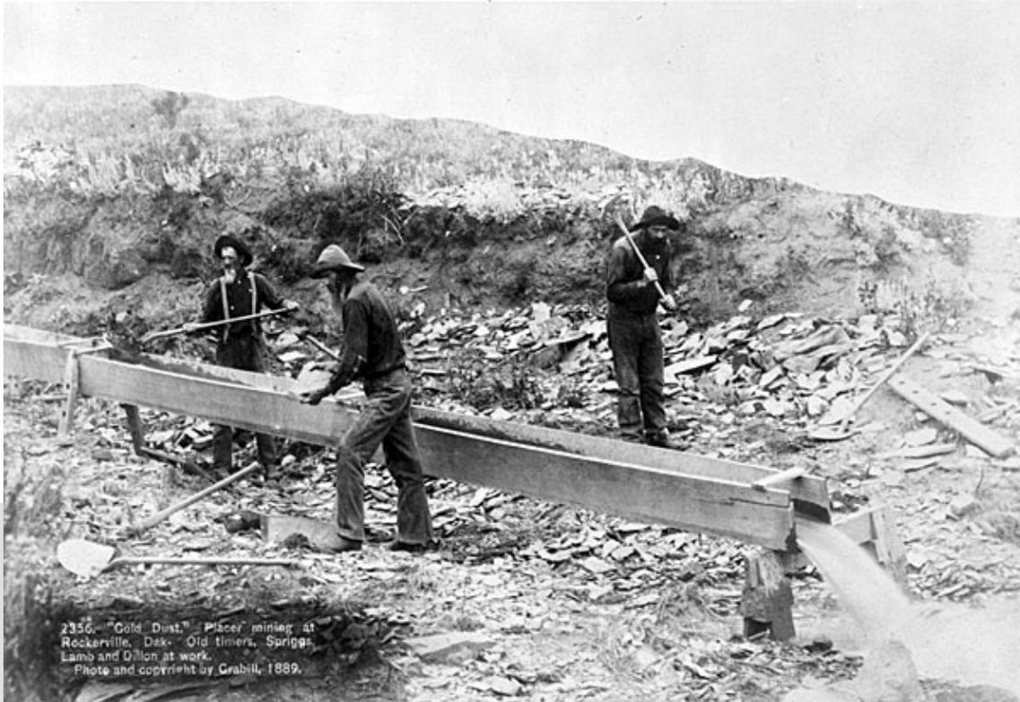
Figure 3.2: A party of miners processes gravel in a small sluice near Rockerville in 1889. The operation is typical of gulch placers. The miners use pick and shovel to break up soil on the far side of the sluice, screen out the large cobbles, and heave the earth into the sluice. Courtesy of the State Archives of South Dakota Historical Society.
