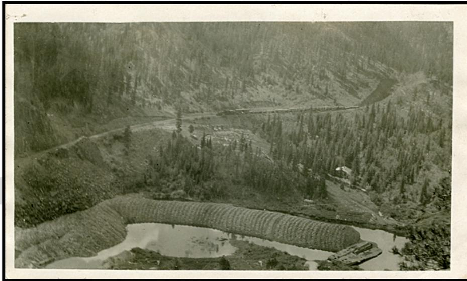
Figure 3.9: Ponds, windrows of tailings, and abrupt contacts between dredge workings and unaltered ground are characteristic of dredge sites. Dredge hulls such as the one at lower right, at Mystic, can be recorded and assessed as individual sites. When combined with the dredged workings, they constitute important mining landscapes. Courtesy of the State Archives of South Dakota Historical Society.
