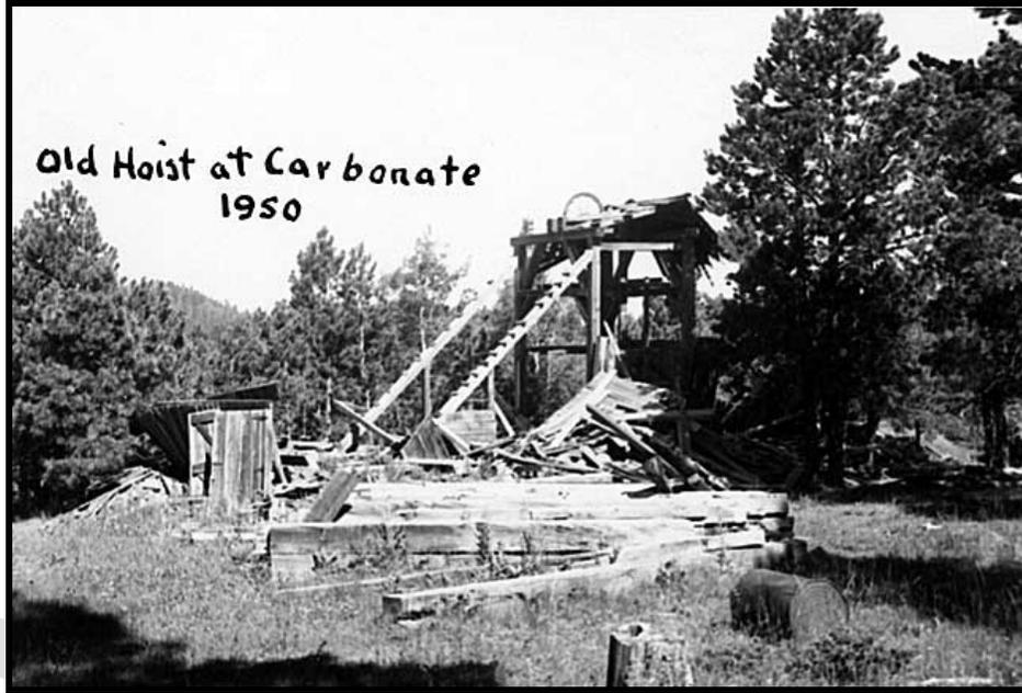
Figure 2.1: The Carbonate Mine, reduced to ruins in this 1950 photo, is an example of a mine site with integrity on archaeological and engineering levels. The headframe is an intact engineered structure, and such resources are rare and important. The collapsed shaft house and other aspects are archaeological features, and they contribute integrity on an archaeological level. Courtesy of the State Archives of South Dakota Historical Society.
