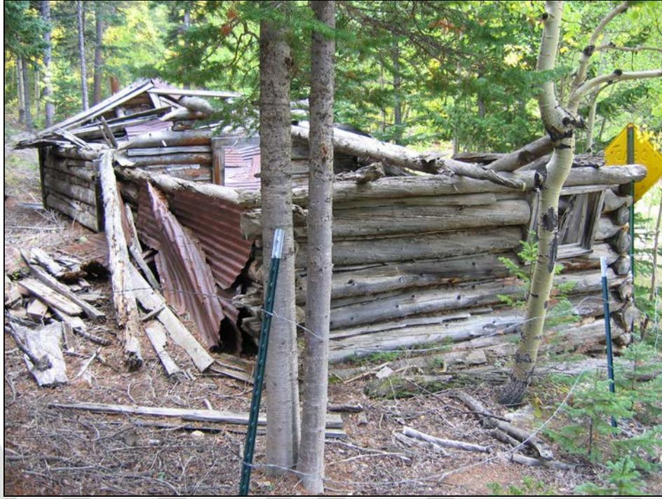
Figure 4.7: When intact, this building was a typical log cabin, but it has decayed into what is currently termed a *cabin ruin*. These types of cabins were a universal form of housing at mines and in towns. Source: Carol Beam, Boulder County Parks and Open Space, Colorado.
