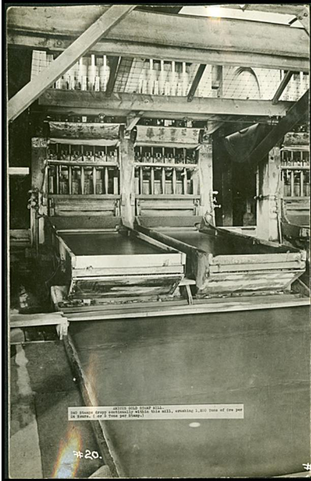
Figure 3.86: The undated photo illustrates amalgamation tables at the Amicus Mill in Lead. The tables, large copper plates coated with mercury, extend outward from the base of stamp batteries. Slurry produced by the stamps flowed over the tables, and the mercury amalgamated with the gold. Courtesy of the State Archives of South Dakota Historical Society.
