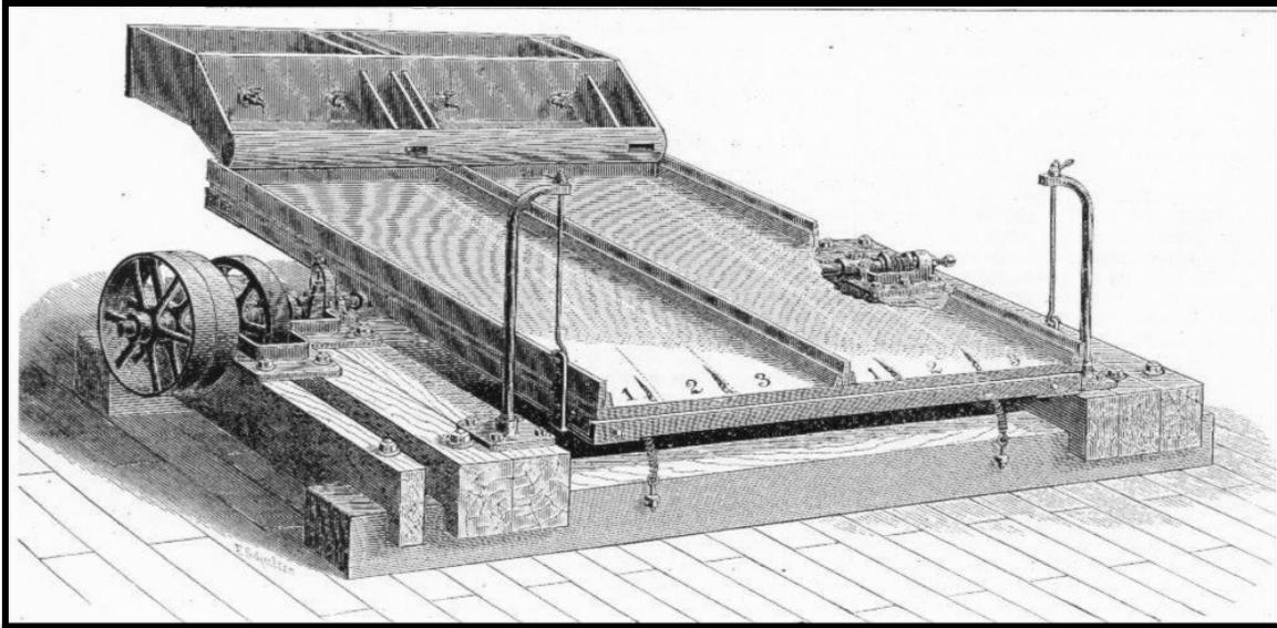
Figure 3.88: Known as both a percussion table and a bumping table, this 1880s apparatus used vibratory action to concentrate finely ground gold and silver ores. Source: *Mining & Scientific Press* 8/9/90, p83.
