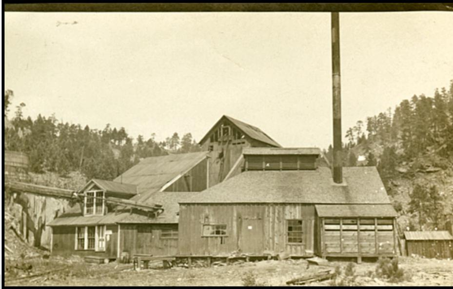
Figure 3.29: The unidentified mine at Deadwood exemplifies a large and complex shaft operation. The building in the foreground with smokestack houses a boiler, and the tall structure behind encloses the mine's headframe and steam hoisting system. Courtesy of the State Archives of South Dakota Historical Society.
