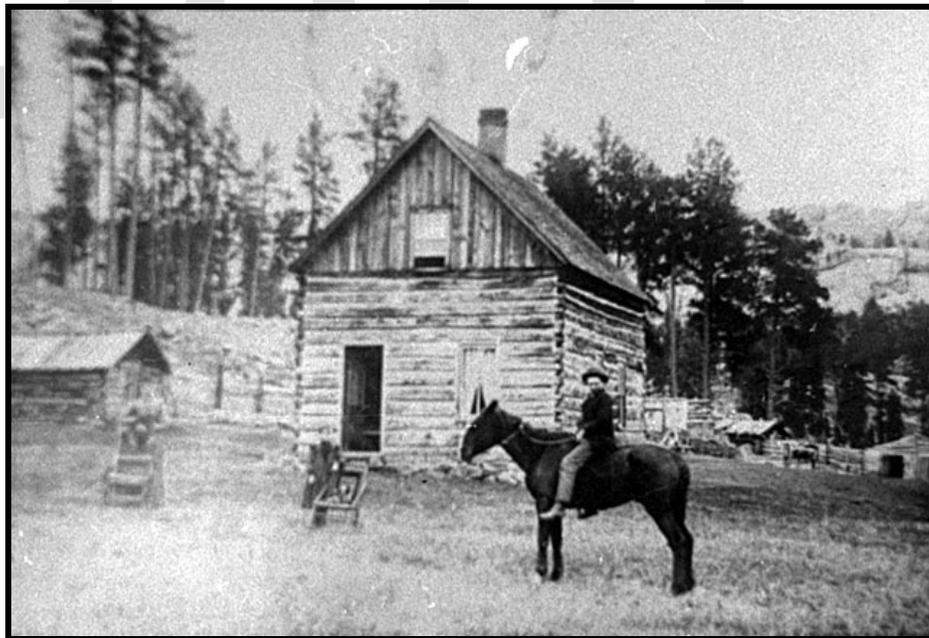
Figure 4.6: This residence in Rockerville exemplifies the log cabins typical of the boom era in the Black Hills. The building is rectangular, vernacular in construction, and one-and-one-half stories high. Lumber, the preferred construction material, began to supersede logs during the 1880s, but logs were common through the 1910s in remote communities. Courtesy of the State Archives of South Dakota Historical Society.
