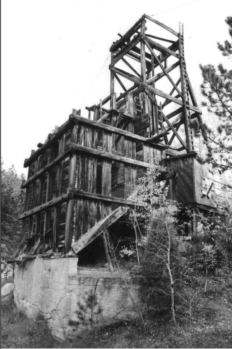
Figure 3.56: Many shaft mines had sloped floor ore bins adjacent to their headframes. Most ore bins stood on the shoulder of a mine's waste rock dump. Source: Eric Twitty.
