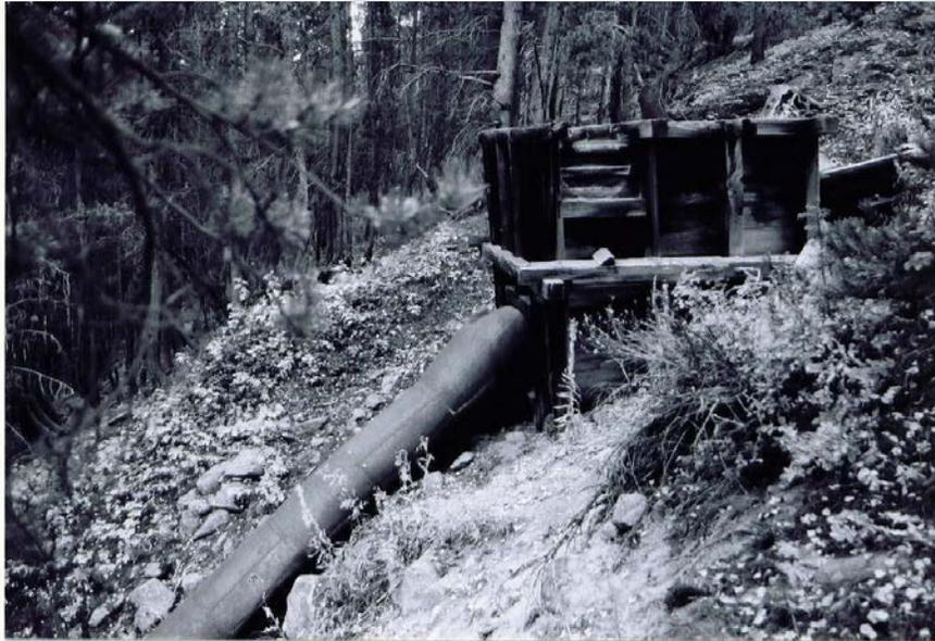
Figure 3.6: The infrastructure for hydraulic mines included components outside of and above the placer workings. A pressure box was a rectangular tank that received water from a ditch and diverted it into a pipeline known as a penstock. The pipeline carried the water under pressure down to monitors in the workings.
