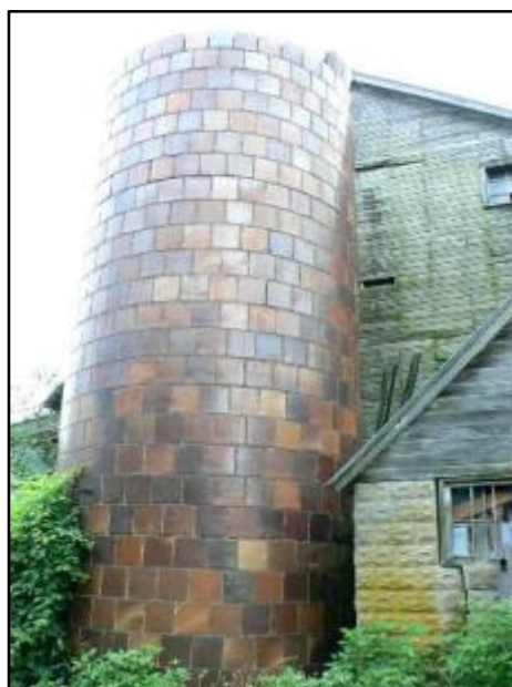
Hollow-tile silo. Photograph by Bill Kibbel, 2004.
