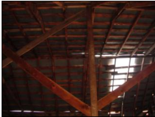
Detail of light truss framing in twentieth century gambrel roofed barn. Photograph by Sean Doyle, 2012.
