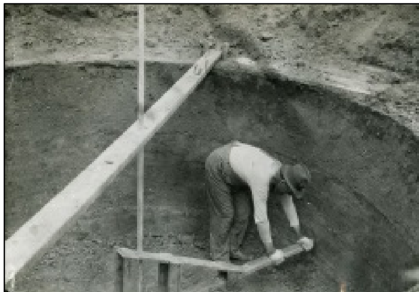
Construction of a pit silo. Haney (1916).
